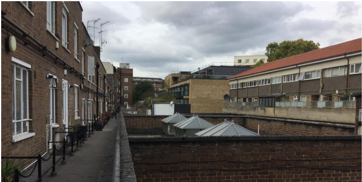
Rear of the application site – looking towards Cervantes Court and Aird House
