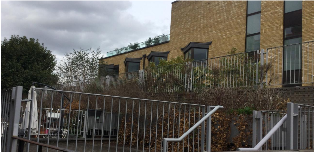
Rear elevation of Aird House
